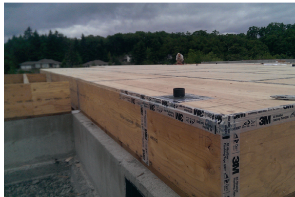
3.3.2 Sheathed and sealed floor framing. BILYEU HOMES INC.
